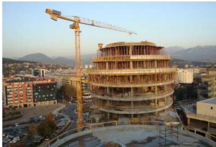
Picture 5: Braces of mezzanine ceilings, PC3
