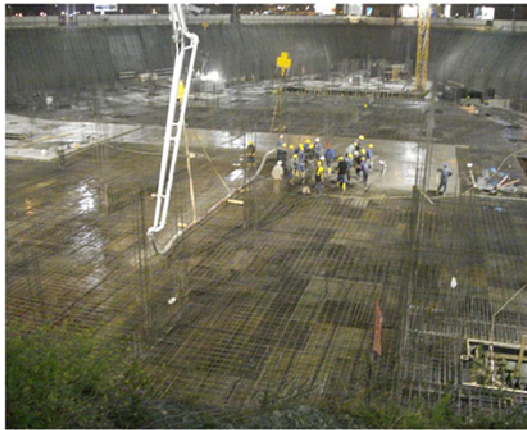
Picture 1: Concreting of base slab
