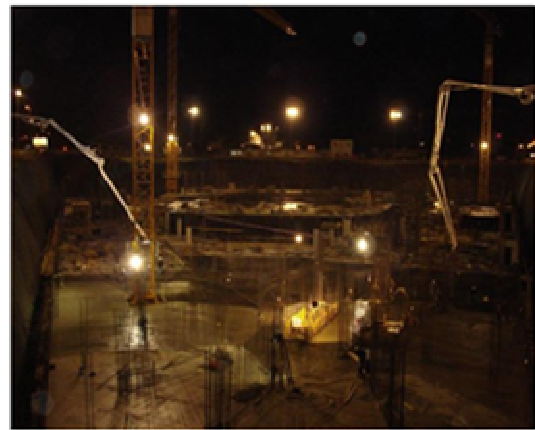
Picture 2 – Night concreting
